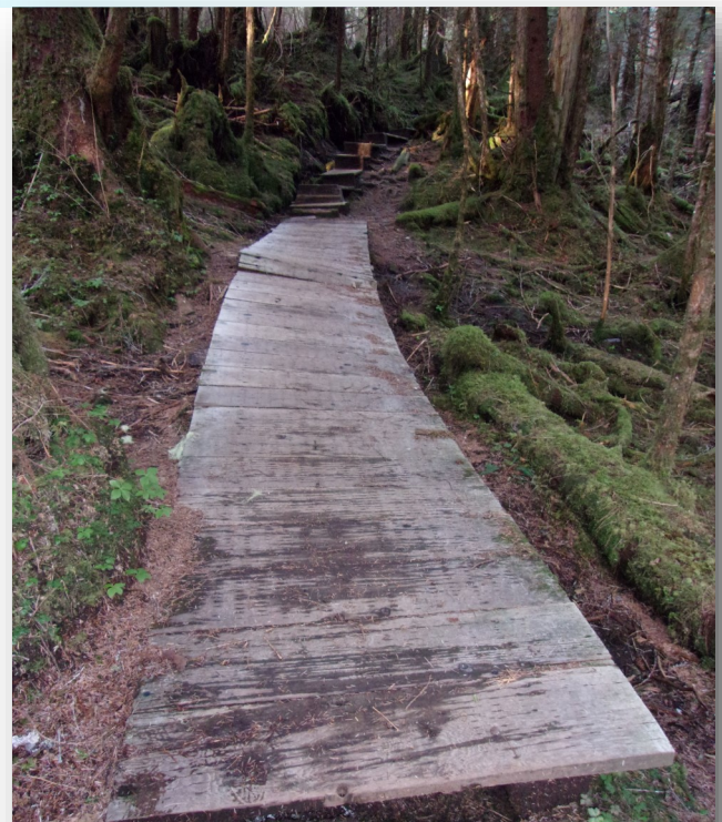
Section of boardwalk to be replaced during this summer's project
