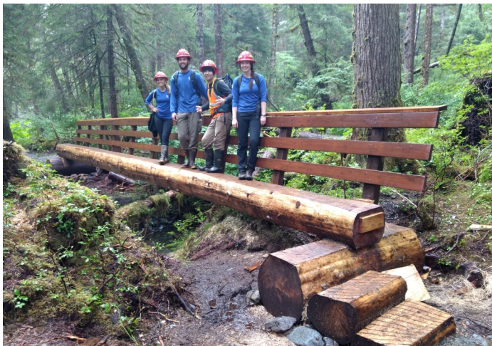
A work crew installing a new log-stringer bridge. This article's photos courtesy of US Forest Service.
